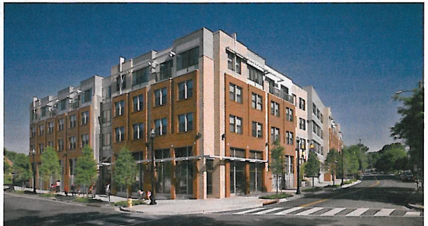
The Shelton earned an honorable mention this year in the metropolitan housing category of the Affordable Housing Tax Credit Coalition's Charles L. Edson Tax Credit Excellence Awards. (Bonstra/Haresign Architects; Photo by Anice Hoachlander)
