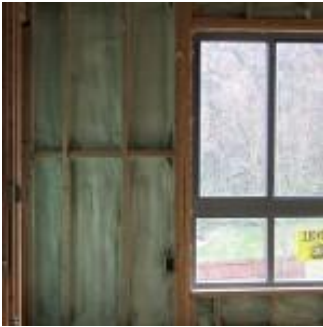
Sprayed in foam insulation
