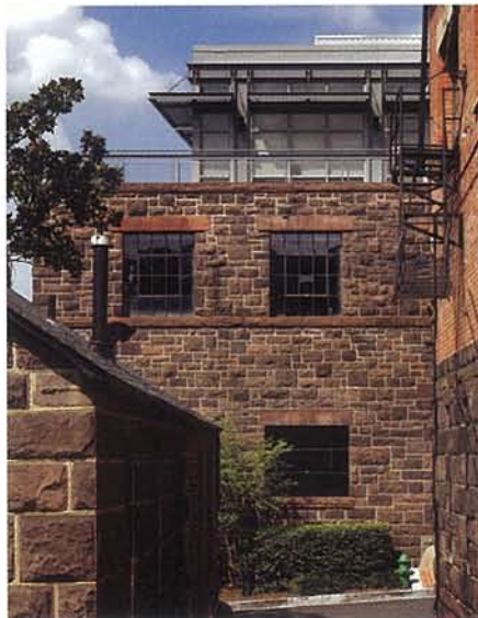
A 1920s automobile warehouse, located immediately adjacent to the C&O Canal in Georgetown, a historic section of Washington, D.C., was converted to a mixed-use project called Caton Walk. The restored building facade and a low and set-back glass-and-steel addition on the roof complements rather than overpowers the existing structure. The detailing of the windows in the new addition echoes the gridded windows in the original edifice.
