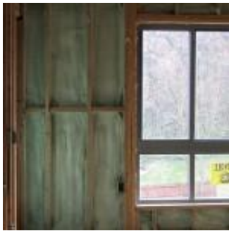
Sprayed in foam insulation
