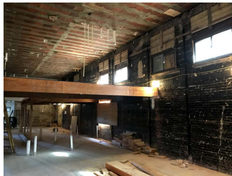
Terrace level lofts under construction; ceiling opened to capture all existing height at clerestory. Loft bedroom inserted within the available height
