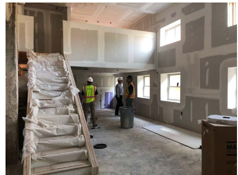
Terrace level lofts under construction; new window wells created to increase daylight access to lower level
