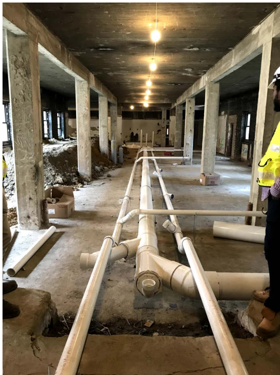
Underslab plumbing before slab infill
