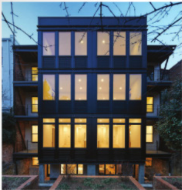
Renovated rear facade, with newly enclosed bays at center.
